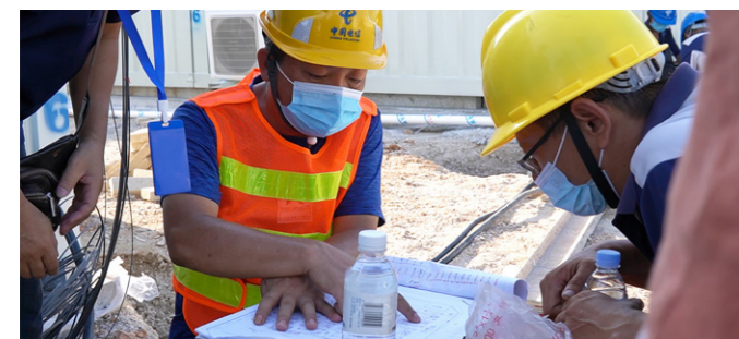
▲ On September 17, 2021, the Zhangzhou Taiwanese Investment Zone in Fujian started the construction of a mobile cabin hospital. The Zhangzhou Branch contacted the management committee of the Taiwanese Investment Zone immediately to understand the network support needs of the isolation sites, and develop the optical cable laying and indoor broadband installation plans. By the early morning of September 22, 2021, all optical cables at the isolation sites had been laid in place, the first batch of 115 sets of broadband had been delivered for use, and the first batch of people for designated isolation had successfully moved in.
